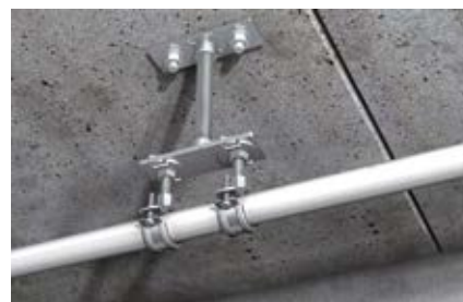
Plastic pipe with fixpoint installation
